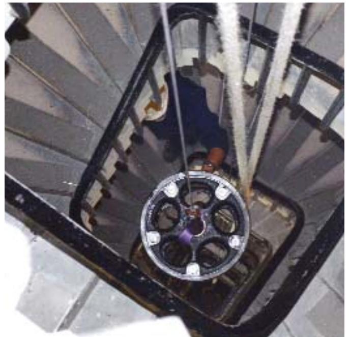
17. The striking barrel being lowered down the stair well.
