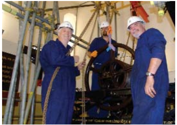
15. Paul, Huw and Ian lifting out the hour striking barrel.
