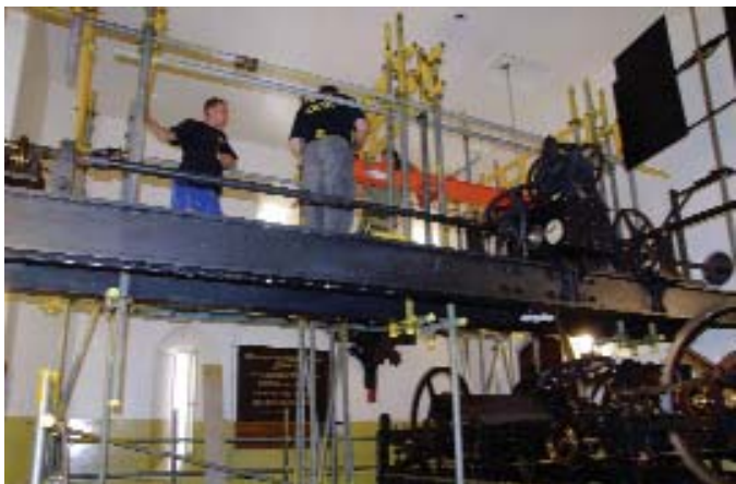
10. Putting up the scaffolding to enable the lifting of heavy parts.
